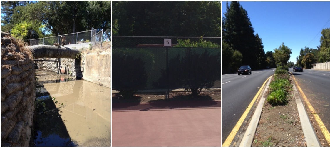
Creek cleaned at Station Ln.
